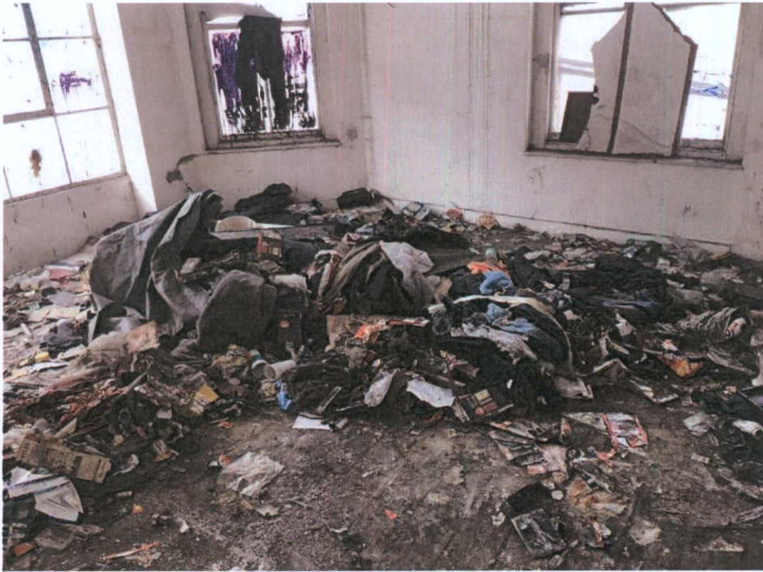
Plate 12.30 Interior view to first floor, facing northwest
