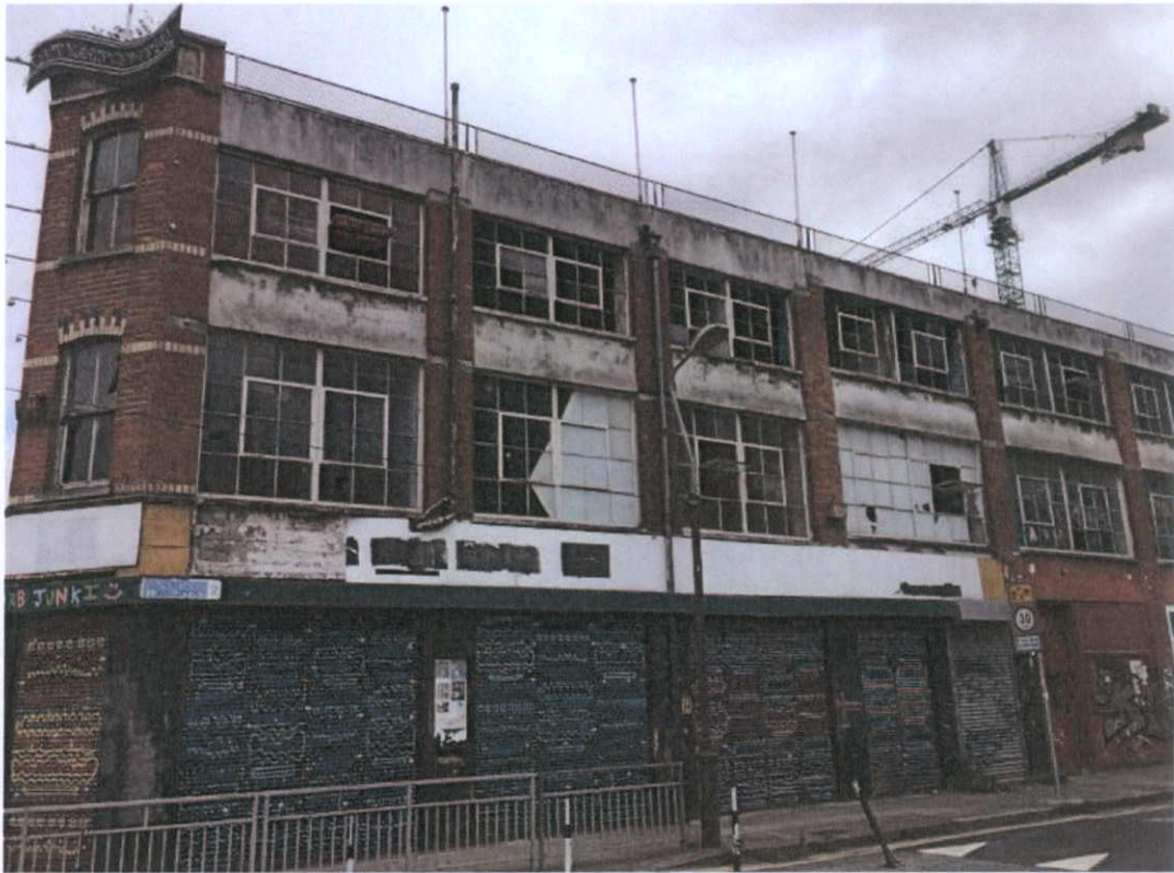
Plate 12.8 Side (west) elevation of art-deco inspired return, facing southeast.
