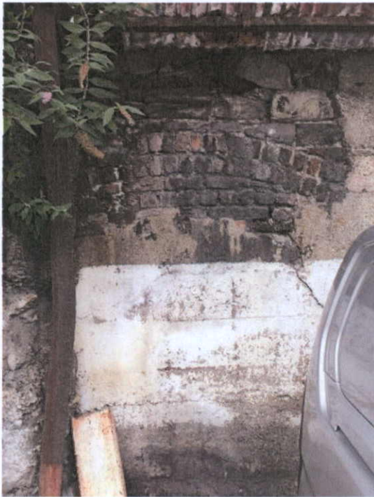
Plate 12.96 View of former opening within eastern boundary wall, facing east
