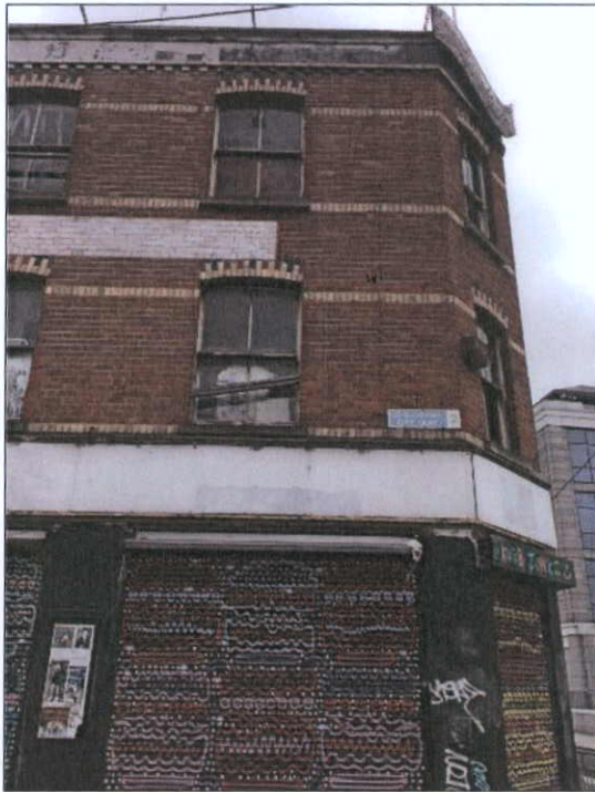
Plate 12.4 Detail to walls and windows to front elevation, facing south.
