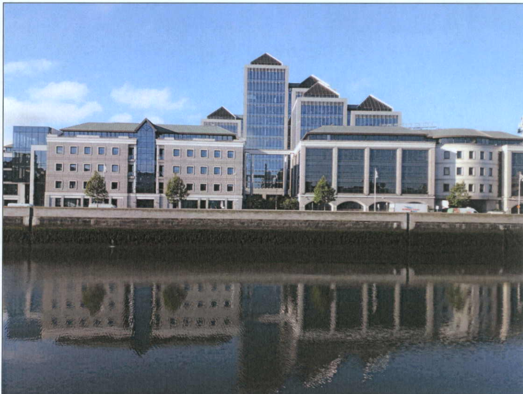
Plate 12.21 George's Quay Plaza with water outflow (centre left) within George's Quay, facing south
