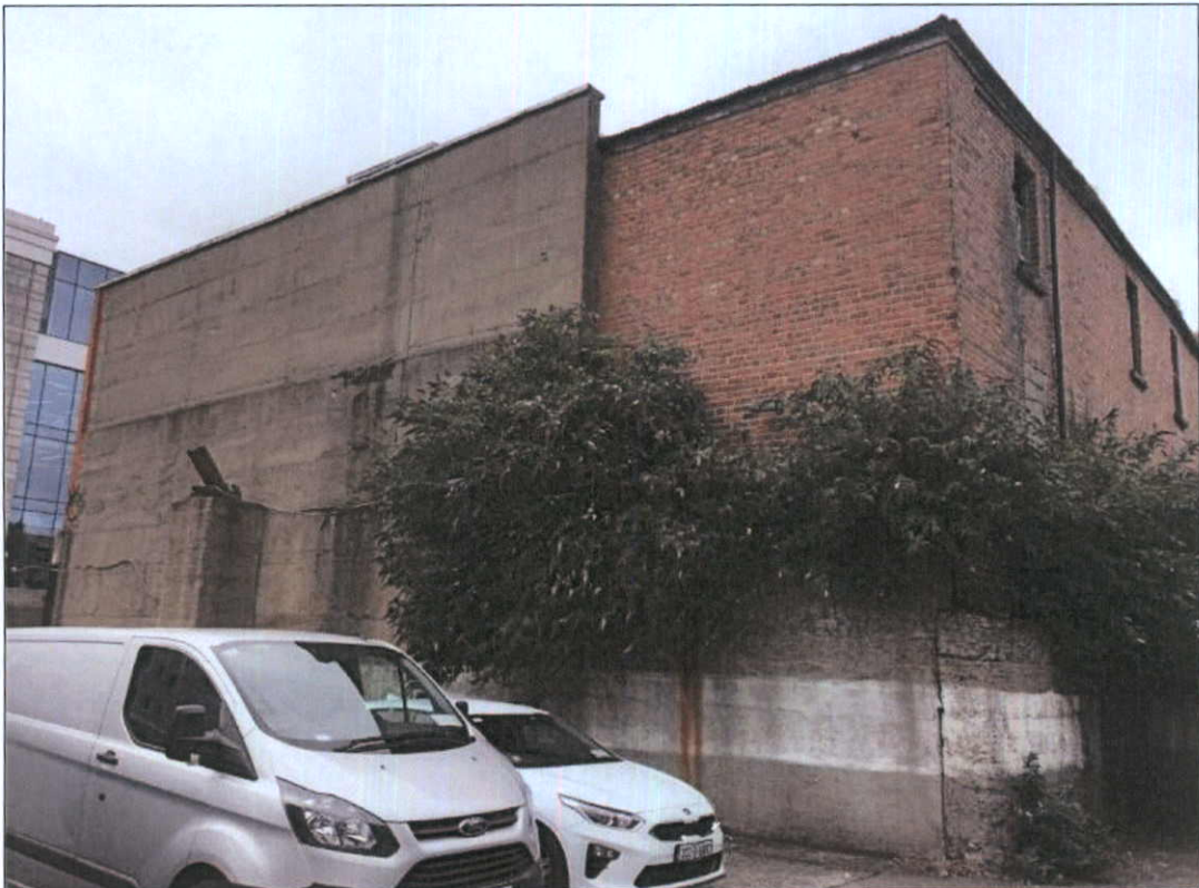
Plate 12.7 Rear (south) elevation, facing northwest.
