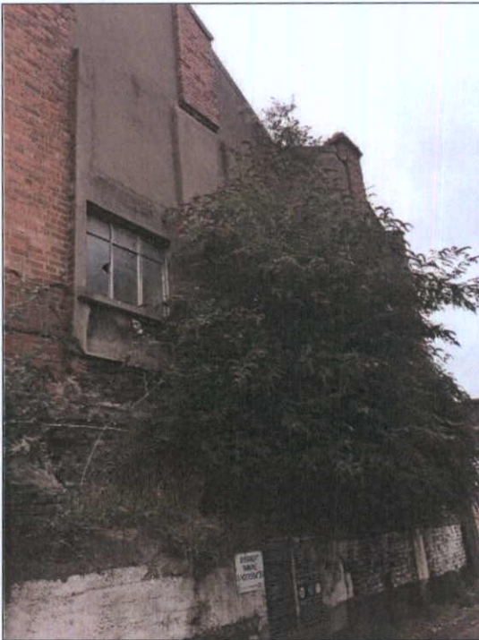
Plate 12.6 Detail of render repairs to side (east) elevation, facing northwest.
